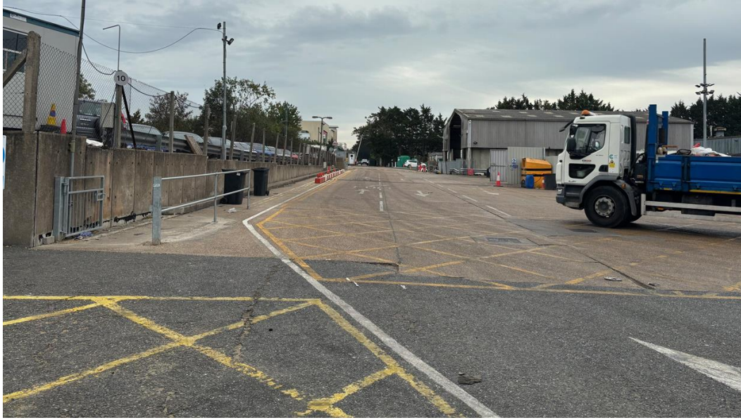
Figure 3 – photo from site towards Baths Road
